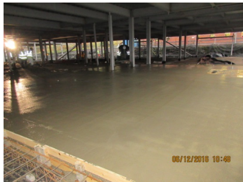
Photograph 9 Concrete placement complete to music department on ground floor
