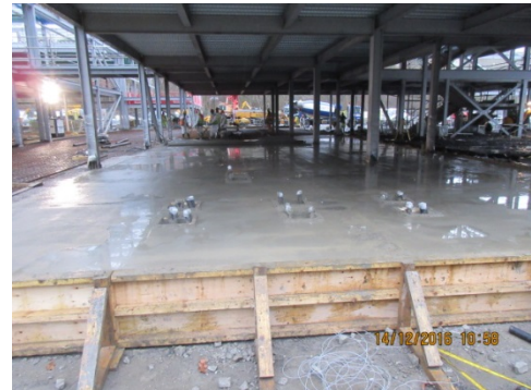
Photograph 8 Placement of concrete to ground floor
