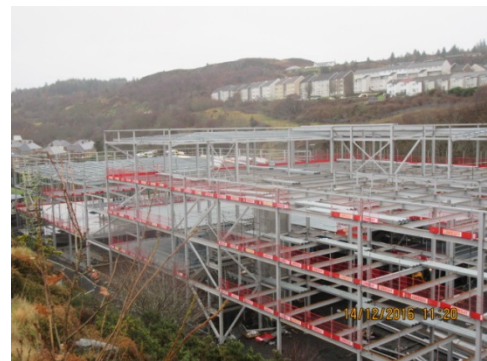
Photograph 2 – View of completed steelwork from rock outcrop
