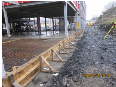
Photograph 7 Perimeter formwork erected for ground floor slab
