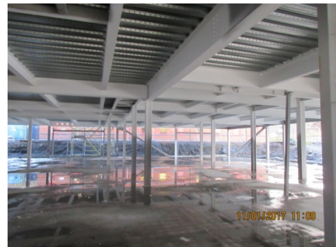
Photograph 10 Intumescent paint applied to internal steelwork
